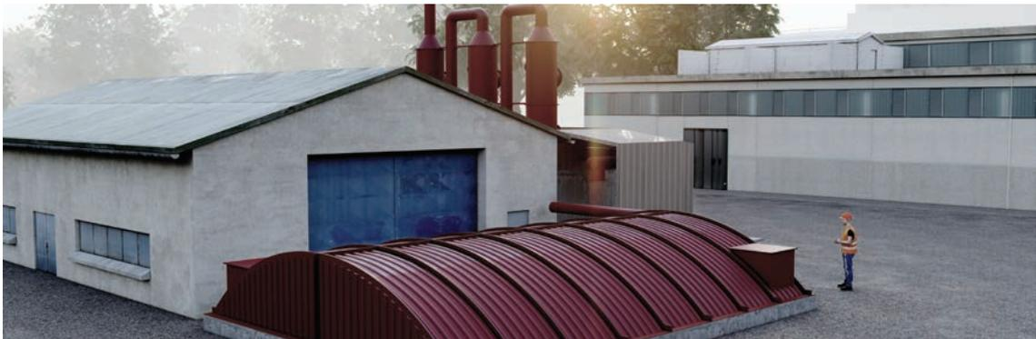
GRP Cover Systems, used to cover sedimentation tanks, sludge tanks and similar open areas in treatment plants, provide both aesthetic and functional advantages. These systems are preferred to prevent odour dispersion, reduce evaporation, direct external rain and snow away from the facility, and create a secure, walkable surface.
