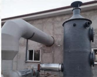
Odour Control Systems are used especially in Wastewater Pumping Stations and Wastewater Treatment Plants to reduce or completely eliminate unpleasant odours. In our company, GRP Scrubber Units, GRP piping and fittings are manufactured for these systems.
