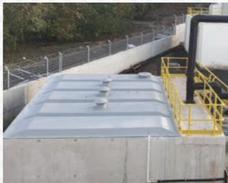
GRP cover solutions are used to safely and aesthetically cover open areas in treatment plants. They prevent odour spread, reduce evaporation and provide protection against external factors. With their lightweight, durable and walkable structure, they offer long-lasting use without maintenance. They can be applied with project-specific dimensions and designs.
